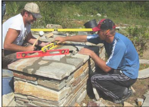
DOUBLE SIDED GAZEBO STONE WALL Random Ashlar and Dry Pac Double Sided Stone Wall With 1-2 inch Stone Cap. -Instructor Iris Lamb and others
