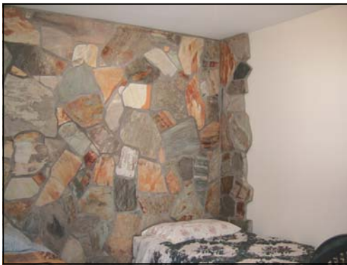
STONE FACING WITH RAKED BACK MORTAR JOINT. - Instructor Iris Lamb
